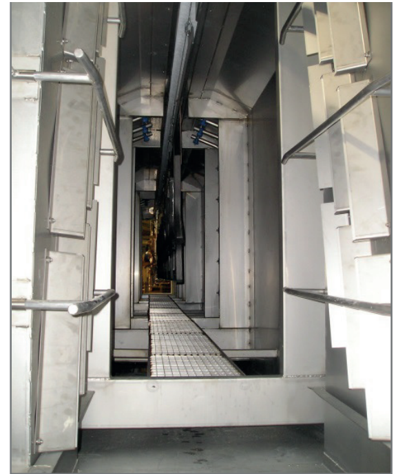
Washing, degreasing, drying and blasting of parts
